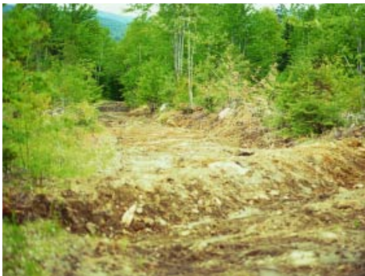
Water bars move water out of the trail onto the forest floor.
