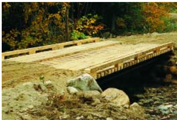
A permanent bridge.
