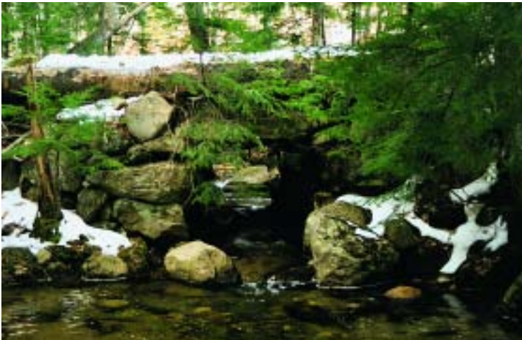
An old stone culvert still functioning.
