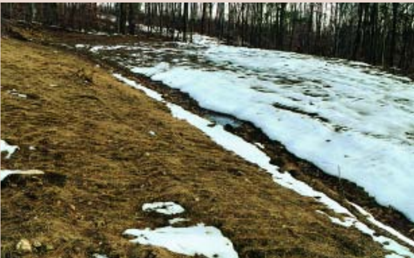
Hay mulch on landing.
