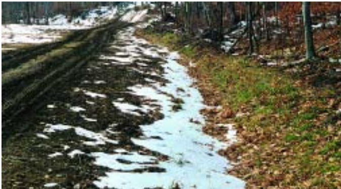
Revegetated road ditches carry water without eroding.
