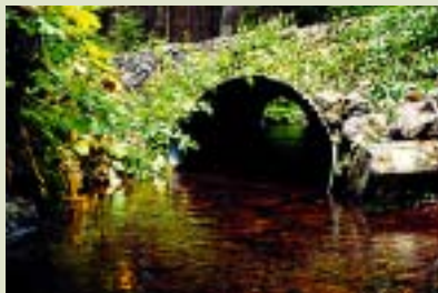
Culvert installed below the streambed level to allow fish passage.
