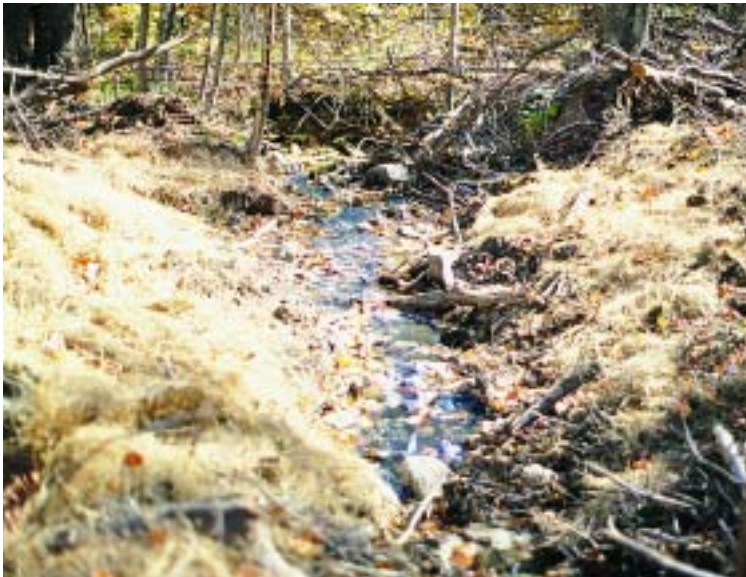
Closeout of a temporary stream crossing.
